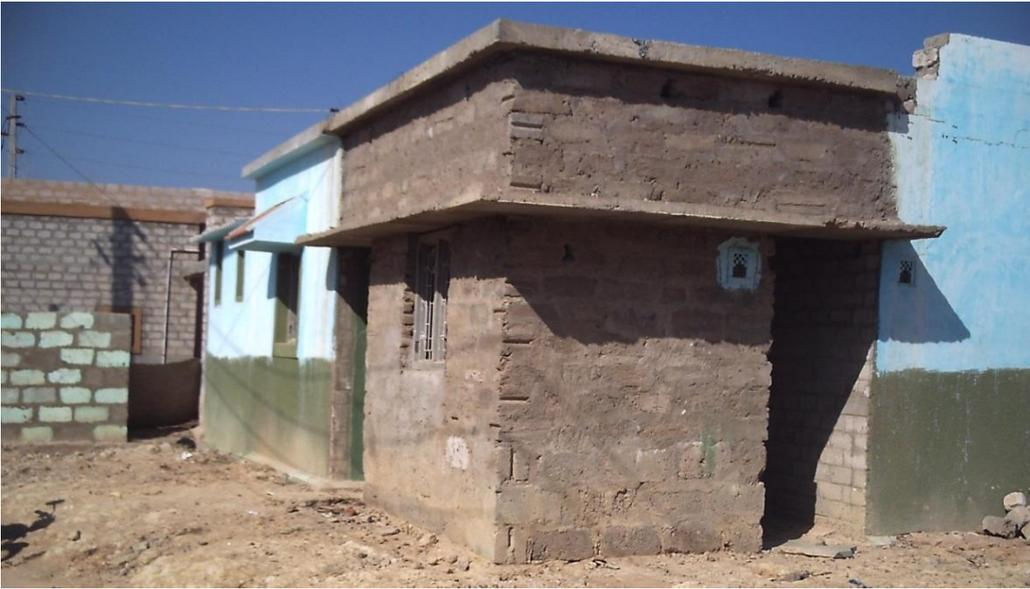
**Fig. 4.28:** Self-built infill construction to the open corner of a Hunnarshālā-designed cluster scheme, built using new materials (SRE block and reinforced concrete). An attempt at design continuity with the new house is evident, along with elements particular to traditional Kutchi houses, such as the small *gokhala*s (niches) to either side of the main door.
