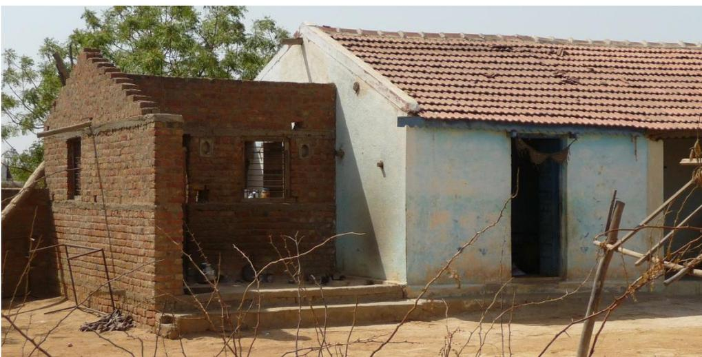
**Fig. 4.71:** A new extension to a reconstructed house which, although incomplete, is already used as a space for cooking. The raft foundation in the foreground implies on-going further development. Note that concrete ring-beam construction has been used, although stabilised rammed-earth blocks have been replaced by more traditional clay bricks.
