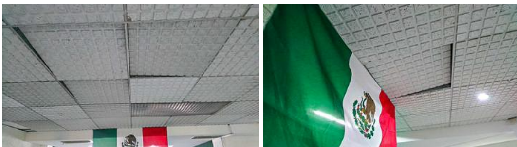
Figure 7.47. Non-structural damage in Condusef Morelos office in Cuernavaca, Morelos (Twitter, 2022n).
