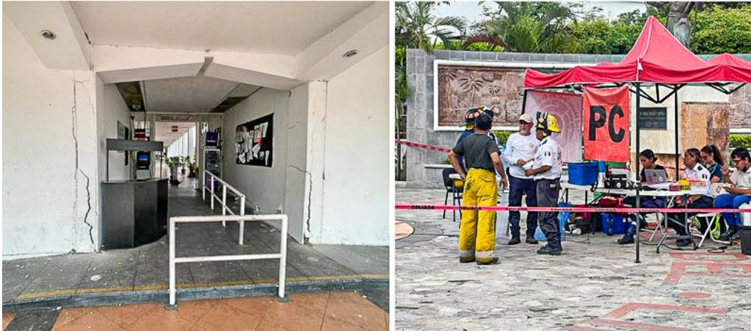
Figure 7.37. Cracks and damaged walls of the “Presidencia municipal de Tecoman” in Michoacán (Diario de Colima, 2022c)
