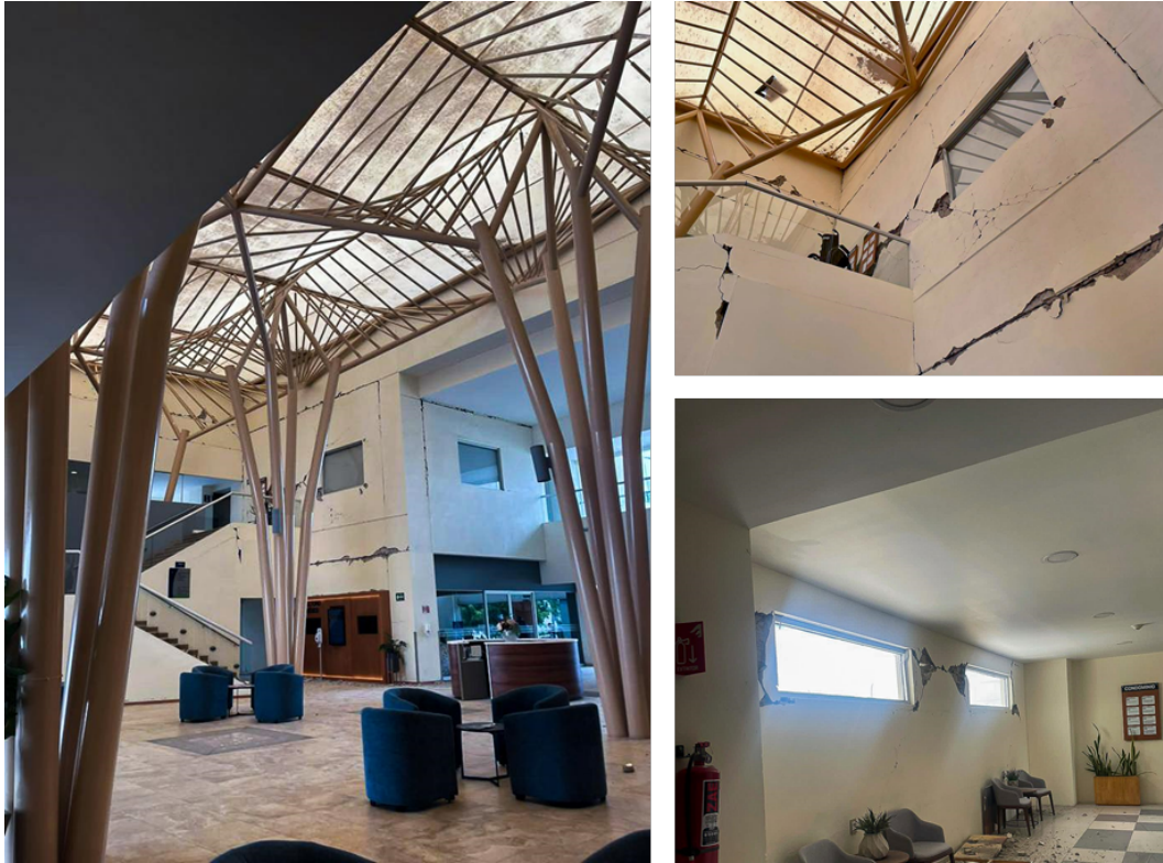
Figure 7.24. Damage to walls of the Hospital Puerta de Hierro in Colima, Colima (Twitter, 2022k).
