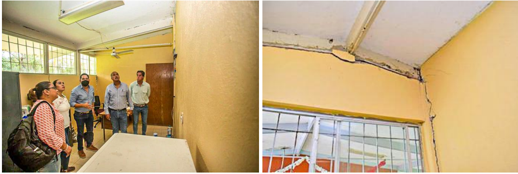
Figure 7.44. Cracked walls of Macario G. Barbosa school in Tecoman, Colima (Twitter, 2022l)
