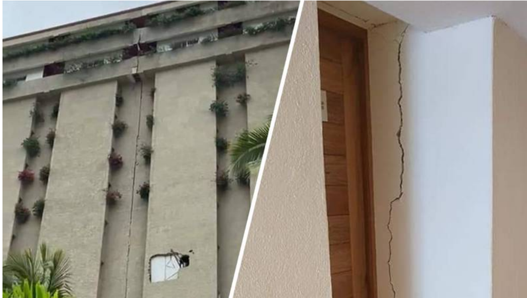
Figure 7.17. Sheraton Buganvillas hotel, Puerto Vallarta, Jalisco. Damage in facades and interior walls. (El Financiero, 2022a).
