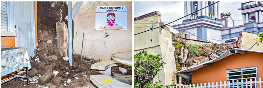
Figure 7.45. Collapsed walls of neighboring structure next to the kindergarten Joseffina Beas in Coquimatlan Colima (Twitter, 2022m)
