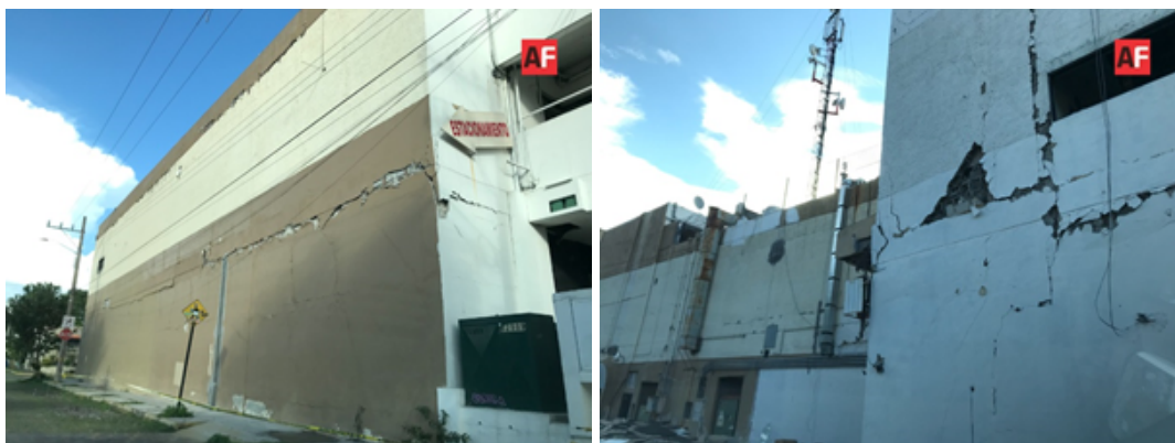
Figure 7.20. Severe cracking on the facade of Plaza Country in Colima, Colima (Facebook, 2022g).
