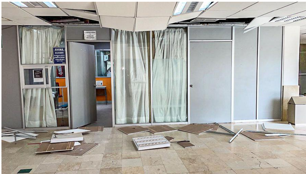
Figure 7.46. Non-structural damage in the Institute of Security and Social Services for State Workers (ISSSTE) in Apatzingan, Michoacán (Twitter, 2022j).
