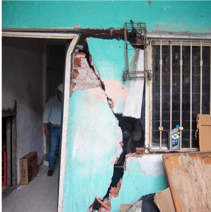
Figure 7.4. Collapsed URM wall in single-family house in Tecomán, Colima (Twitter, 2022f).
