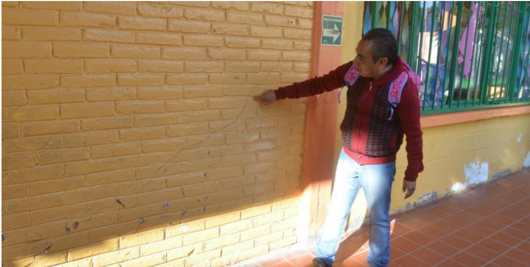
Figure 8.18. Diagonal cracking in masonry infill wall in a school. (La Razón, 2022b)
