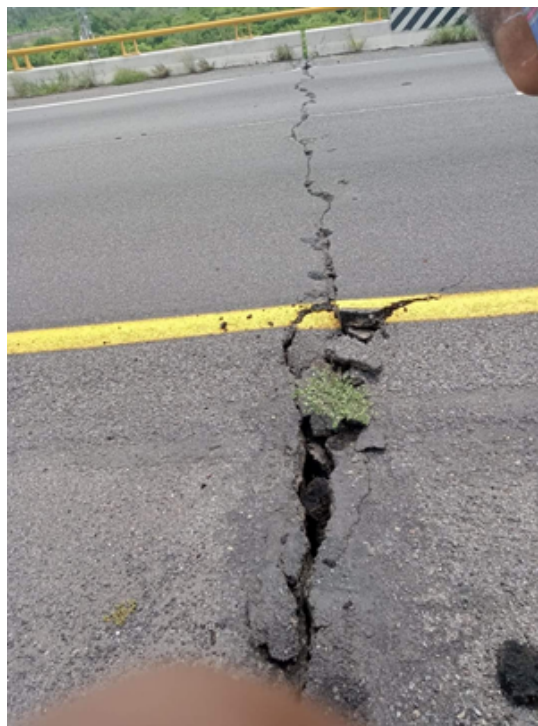
Figure 7.59. Damage at a joint in the Armería bridge located on the federal highway Colima-Manzanillo en Tecmán, Colima (Facebook, 2022k).
