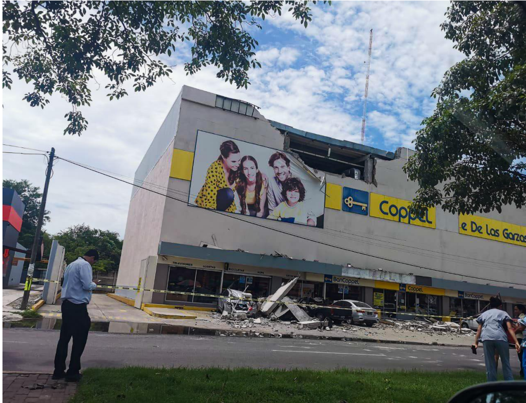
Figure 7.15. Out-of-plane wall failure in the Coppel store at Valle de las Garzas in Manzanillo, Colima which resulted in one fatality (Twitter, 2022e).
