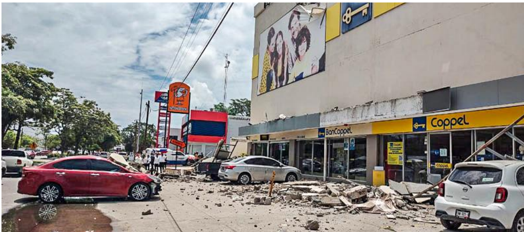
Figure 7.14. Out-of-plane wall failure in the Coppel store at Valle de las Garzas in Manzanillo, Colima (Diario de Colima, 2022b)
