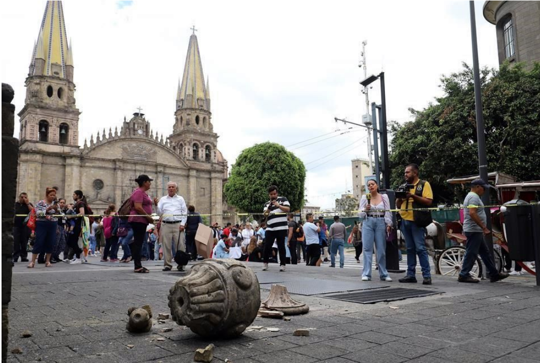
Figure 7.31. Detachment of an ornamentation in the La Merced Church in downtown Guadalajara, Jalisco (Reforma, 2022)
