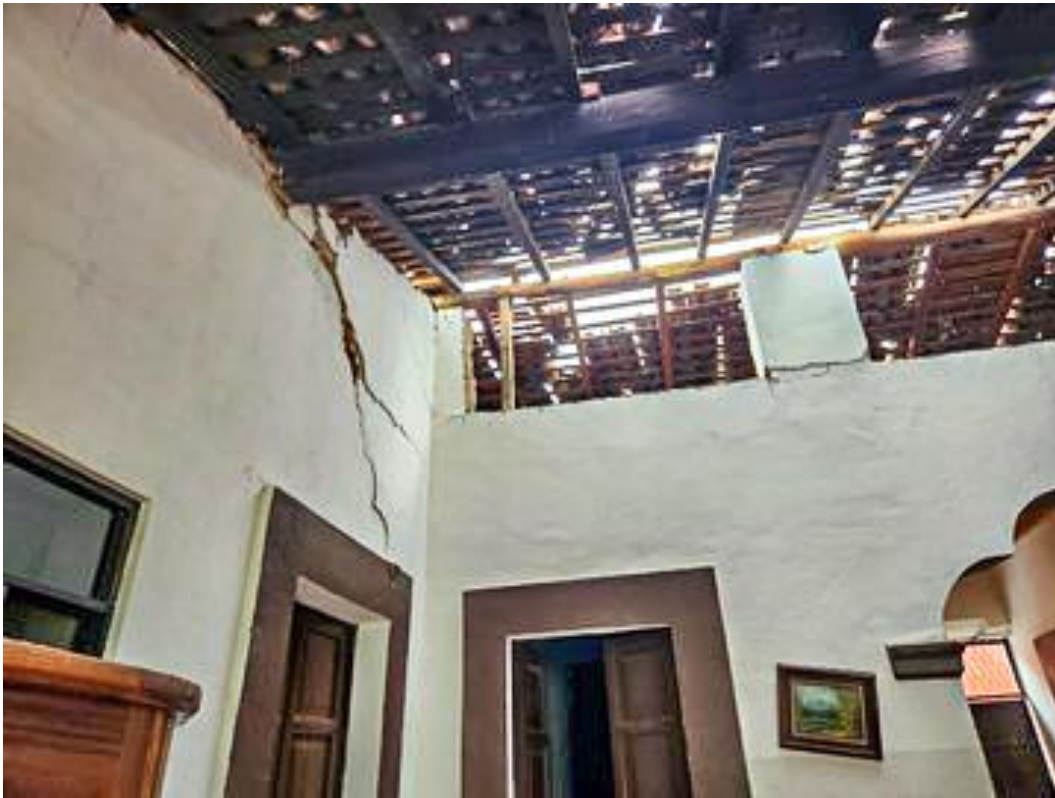
Figure 7.28. Damage to roof and walls in historical buildings in Coalcomán, Michoacán (Twitter, 2022w)
