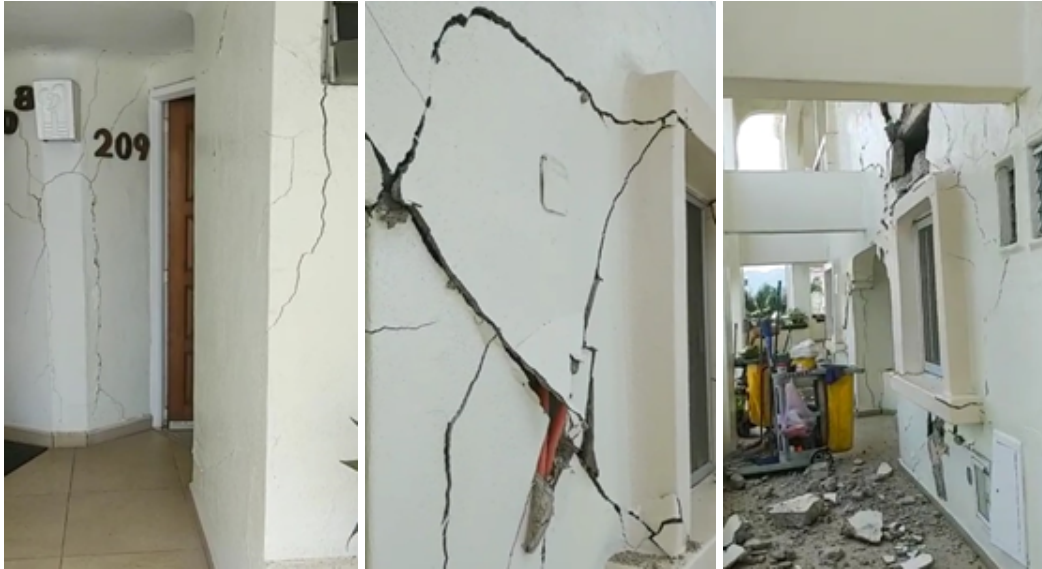
Figure 7.19. Severe wall damage in Gran Pacífico Hotel in Manzanillo, Colima (Colima Noticias, 2022).
