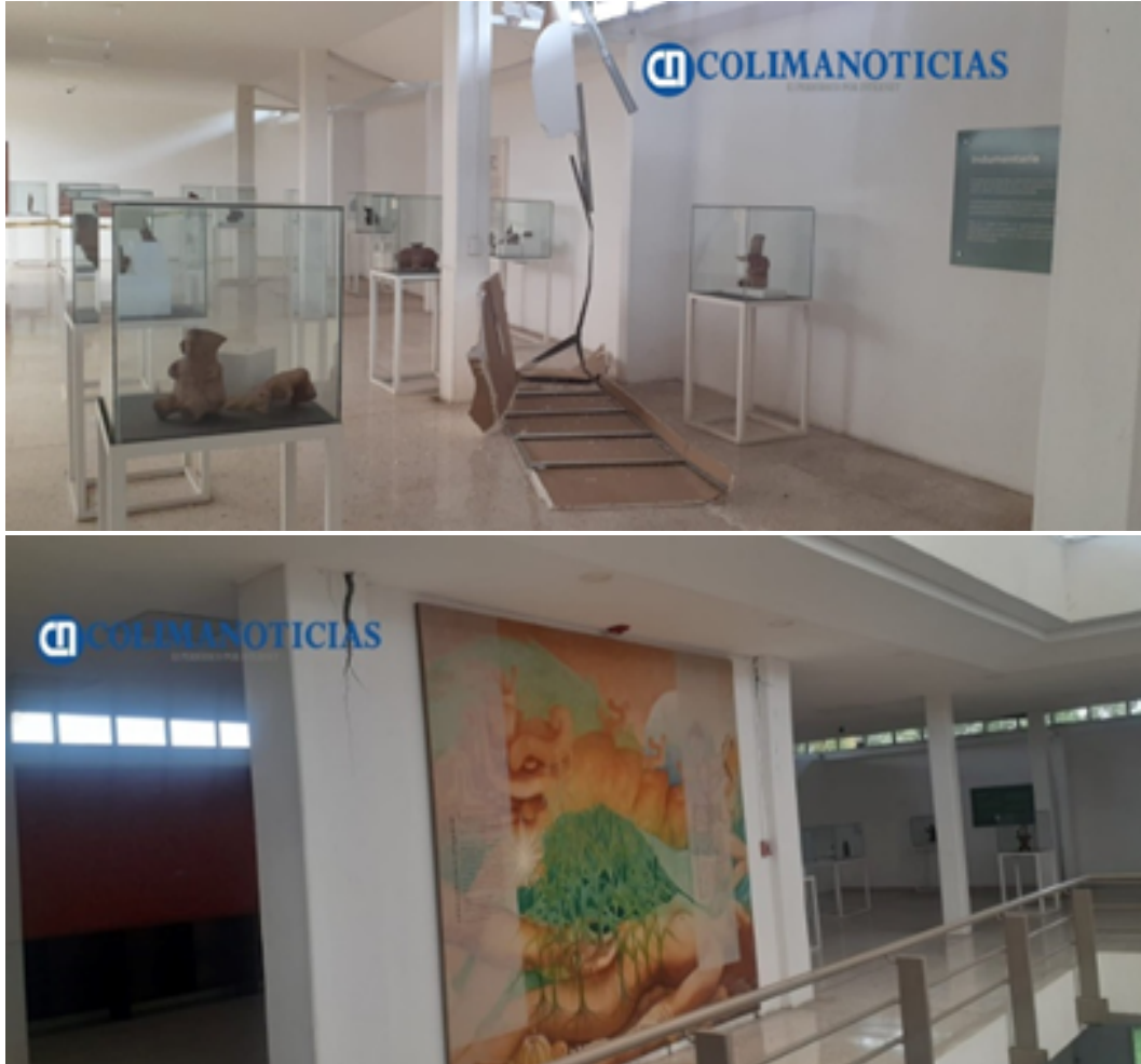
Figure 7.40. Damage to ceilings and severe cracking on walls in the Culturas del Occidente Museum in Colima, Colima (Facebook, 2022p)
