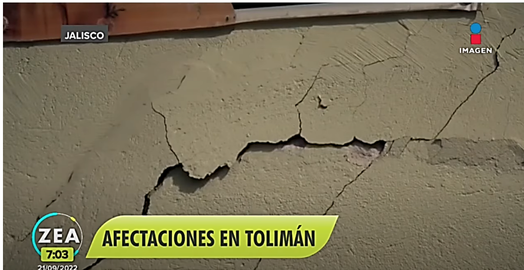
Figure 7.6. Cracking wall in a unreinforced masonry house in Tolimán, Colima (Imagen Noticias, 2022)
