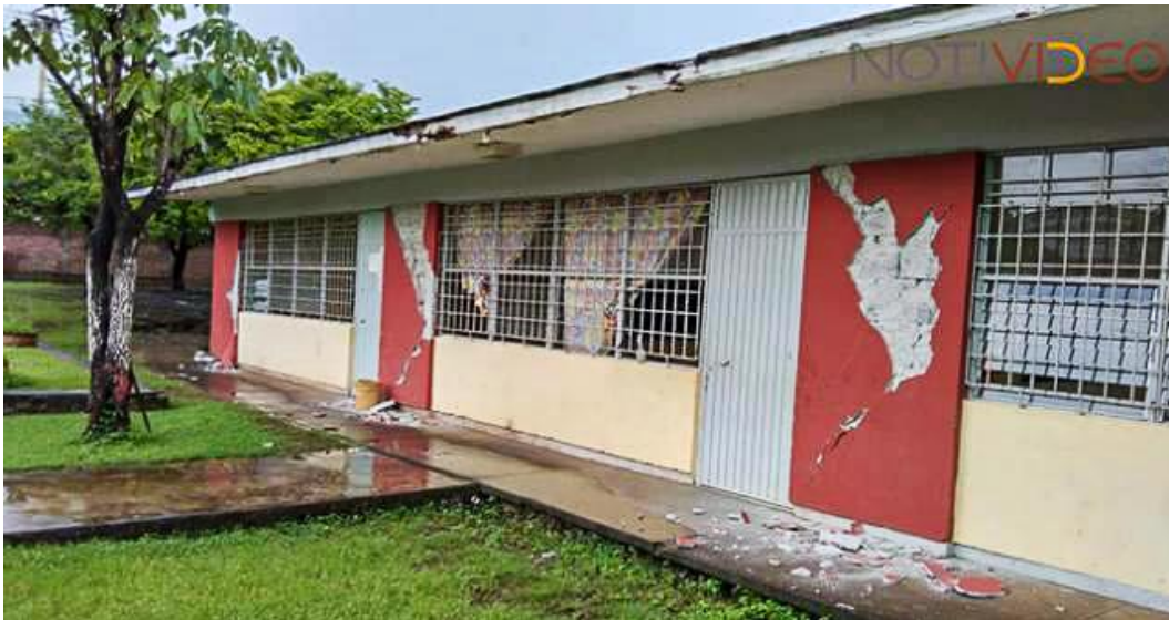
Figure 7.43. Cracked walls of a school in Coalcoman, Michoacán (Notivideo, 2022).
