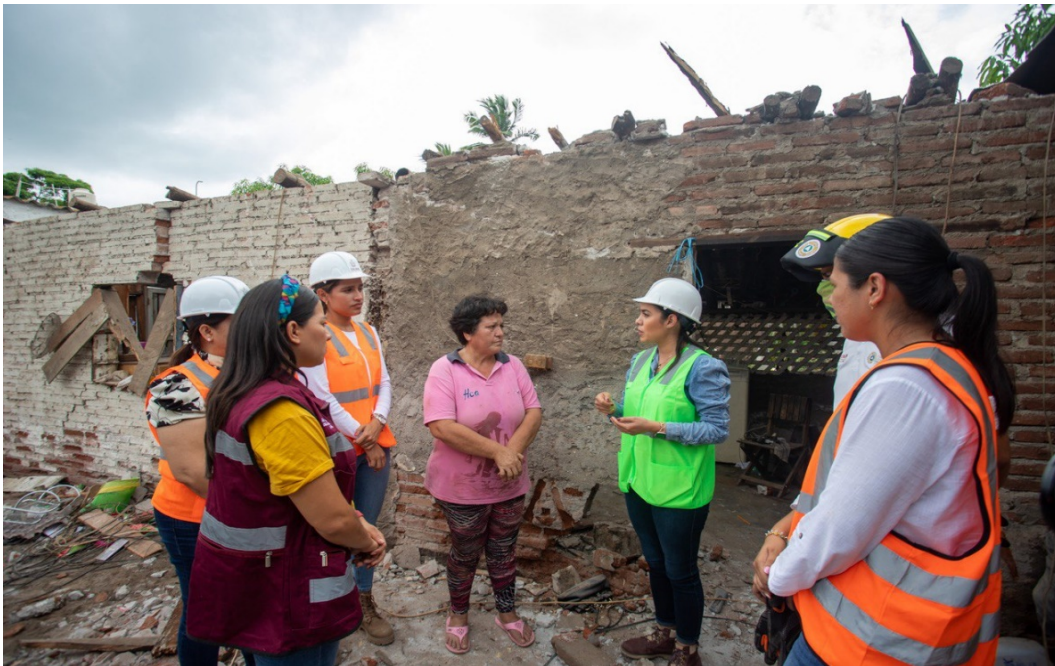
Figure 7.5. Single-family building in Armería, Colima with collapsed wooden roof. The state governor visited affected regions. Many single-family buildings are made of unreinforced masonry, which are highly vulnerable to ground motions. This type of damage is typical in the affected regions (Facebook, 2022c)
