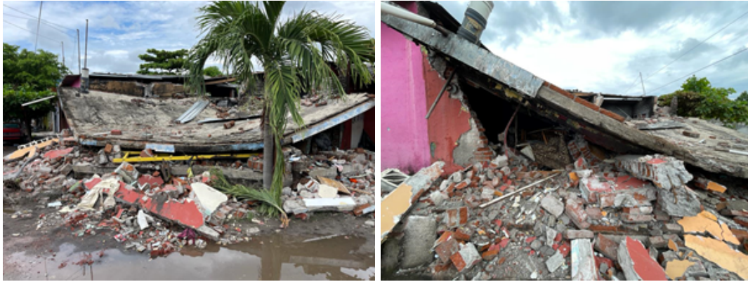
Figure 7.8. Total collapse of a reinforced concrete single-family building with masonry infill walls in San Isidro, Tecomán, Colima (Facebook 2022d)
