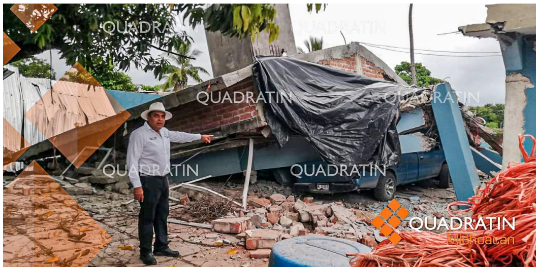
Figure 7.7. Total collapse of a reinforced concrete single-family building with masonry infill walls in San Vicente, Michoacán (Twitter, 2022c).
