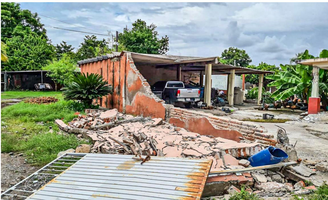
Figure 7.3. Collapsed URM wall in single-family buildings in Morelia, Michoacán (Quadratin, 2022b).
