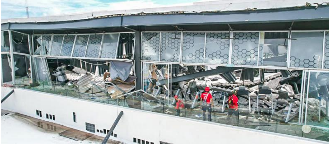
Figure 7.13. Collapsed roof in Plaza Punto Bahía in Manzanillo, Colima (Diario de Colima, 2022a)
