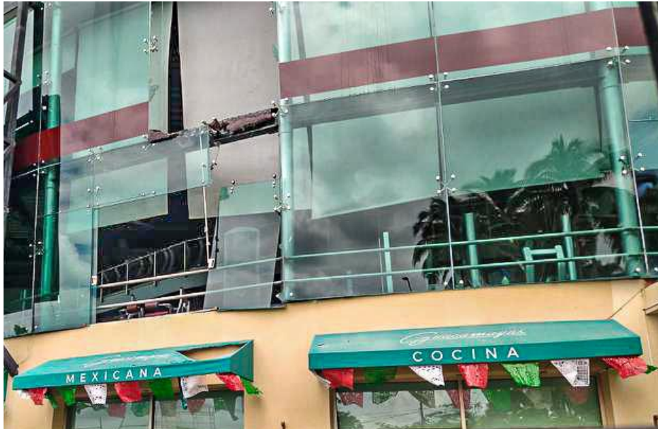
Figure 7.48. Non-structural damage of the mall in Colima, Colima (Publimetro, 2022).
