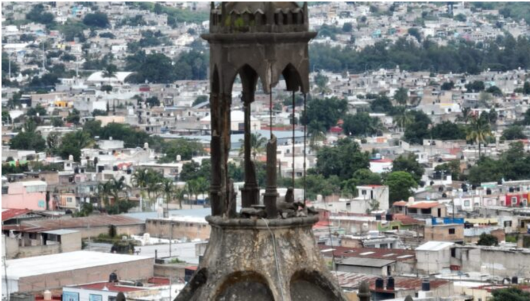
Figure 7.33. Damage at the upper portion of the bell tower in the Asunción Maria Cathedral in Tepic, Nayarit (Meridiano.mx, 2022)
