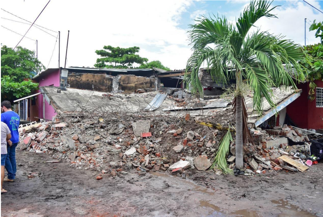
Figure 7.2. URM single-family house completely collapsed in Coalcoman, Colima (PBS, 2022).
