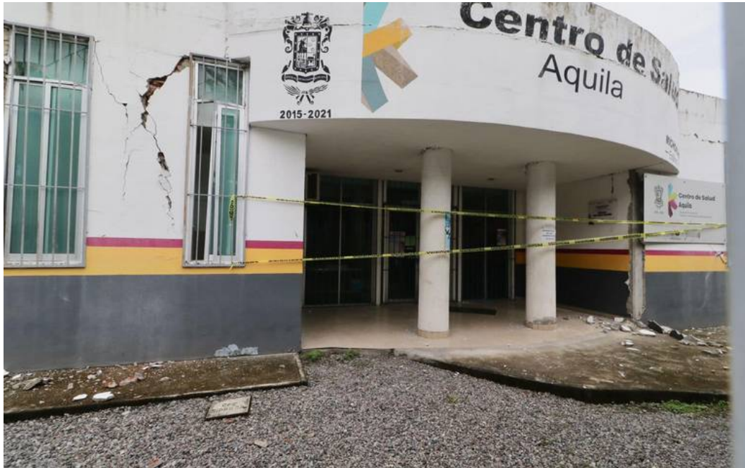
Figure 7.23. Health center at Aquila, Michoacán. The building was evacuated due to structural damage. (El Sol de Morelia, 2022b)
