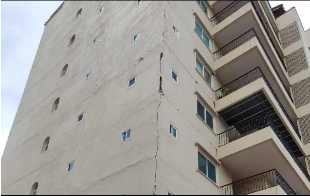
Figure 7.10. Tres Mares Condominium in Puerto Vallarta, Jalisco. Only nonstructural damage was observed and mainly occurred in facades, tiles and ceilings (Informador.Mx, 2022).
