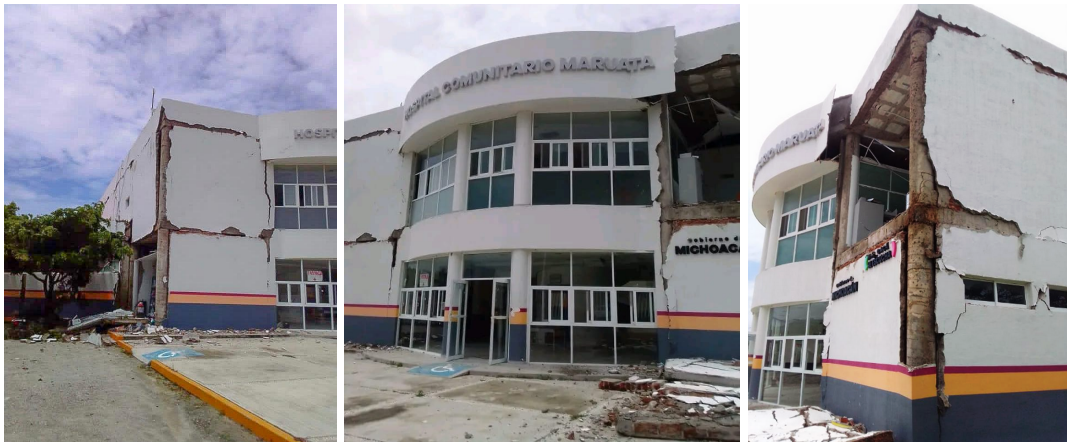
Figure 7.22. Exterior of the Maruata Hospital, Maruata, Michoacán after the earthquake: Masonry facade collapse, exposing significant steel corrosion in columns (Twitter, 2022g)
