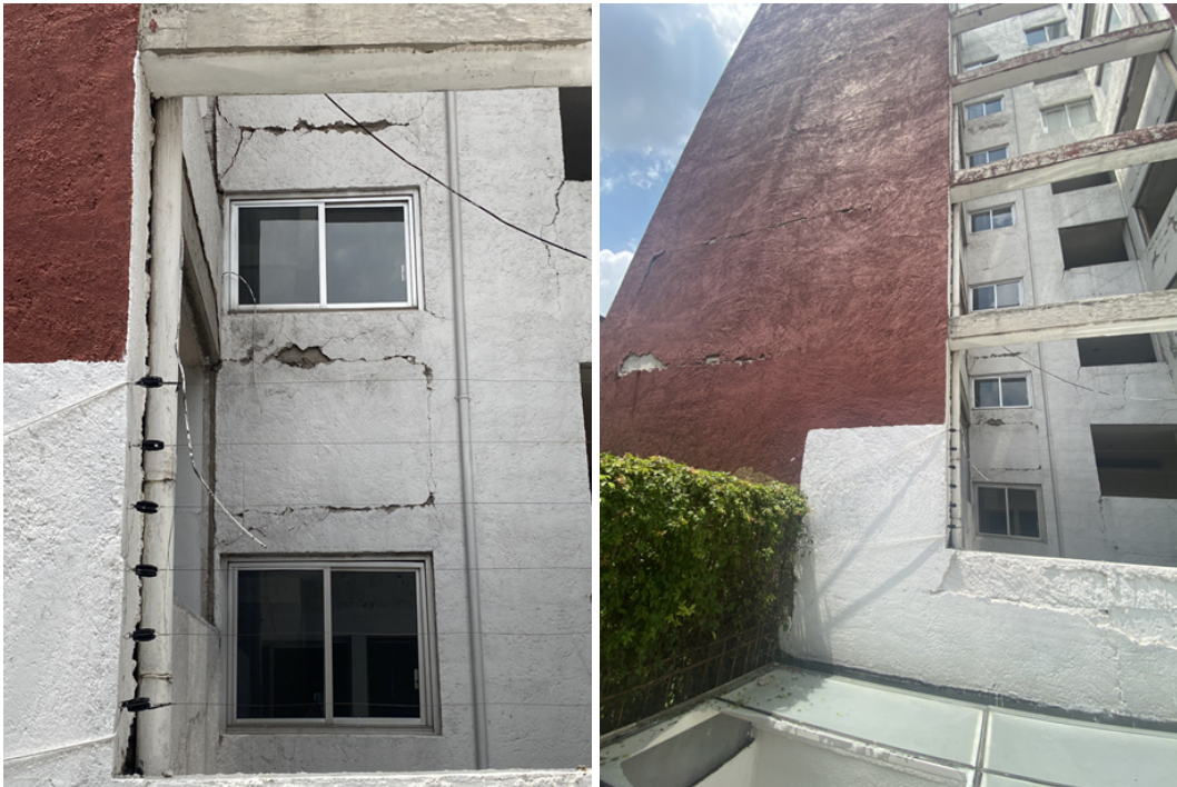
Figure 8.13. Building located at Canal de Churubusco # 351 with some cracks and damage in the facade (Twitter, 2022v).
