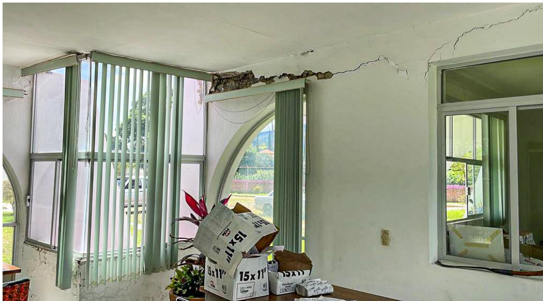
Figure 7.41. Cracked walls in the school of Jiquilpan, Michoacán (Cambio de Michoacán, 2022).
