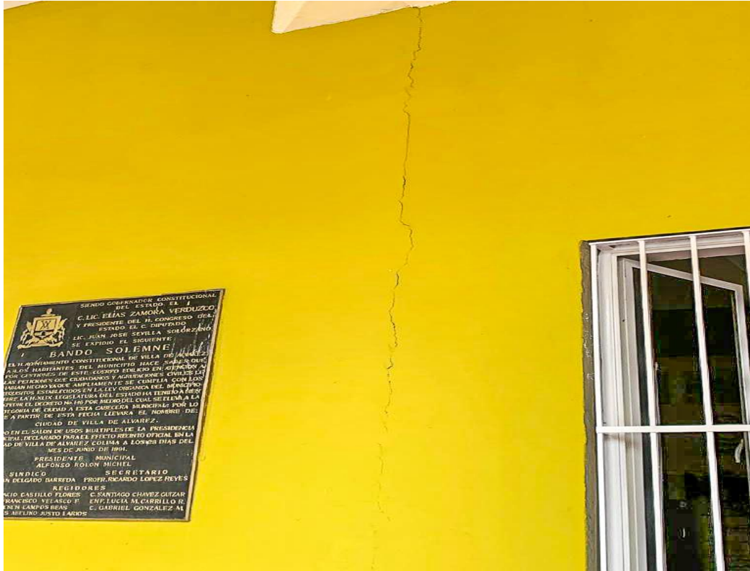
Figure 7.38. Minor cracks in walls of the government building in Villa Alvarez, Colima (Archivo Digital, 2022)
