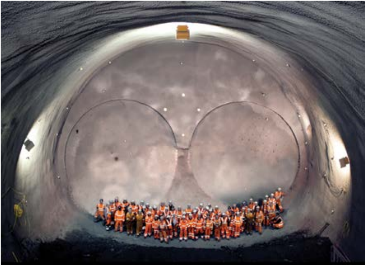
Completion of eastbound cavern at Stepney Green shaft.
