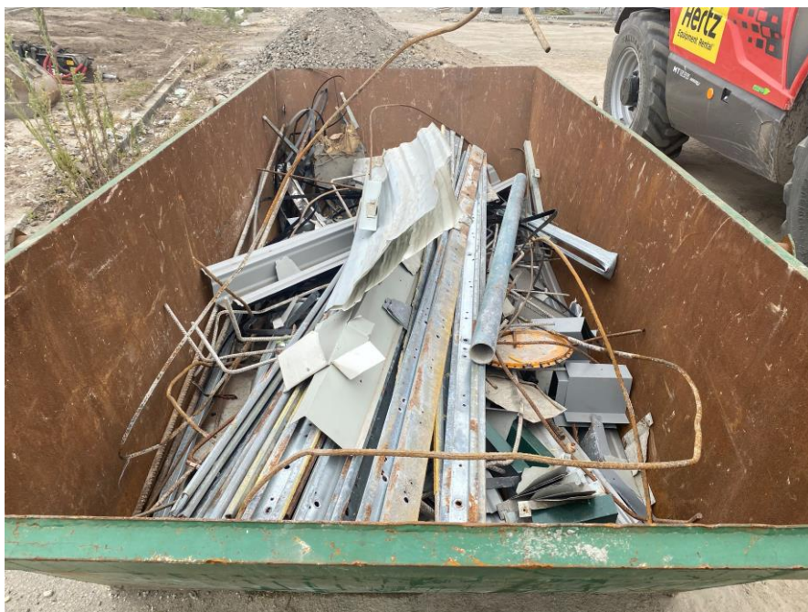
Figure 10. Sorting of metal waste in construction site Source: Taken by project team at site, 2021
