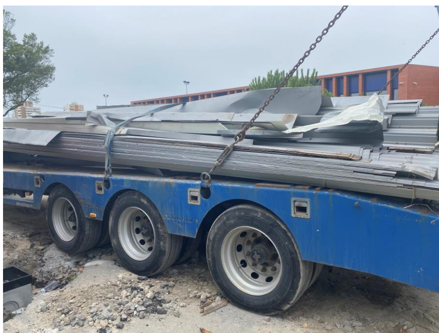
Figure 6. Waste metal sheet sorted in the construction site of the school Source: Taken by project team on site, 2021
