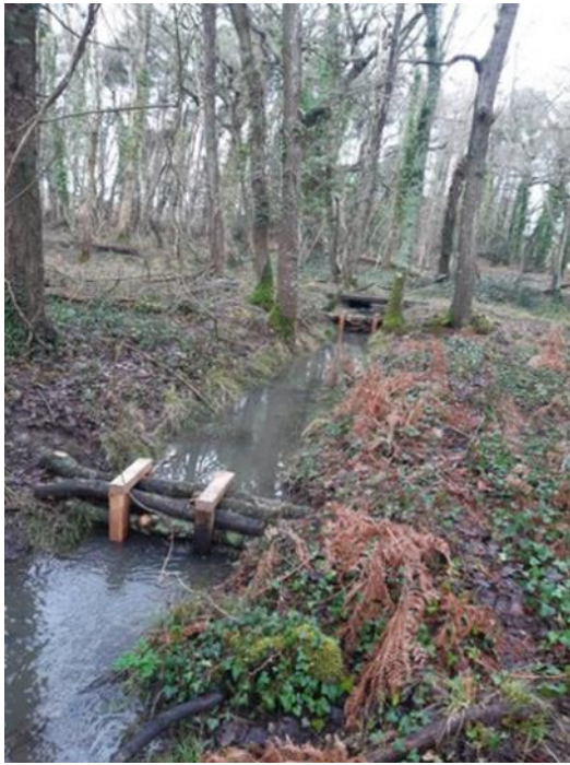
Timber logs from the estate have been utilised to create a secure leaky dam structure in channel to intercept nutrients and sediments. These installations also slow the flow backing up water increasing the potential for natural processes.
