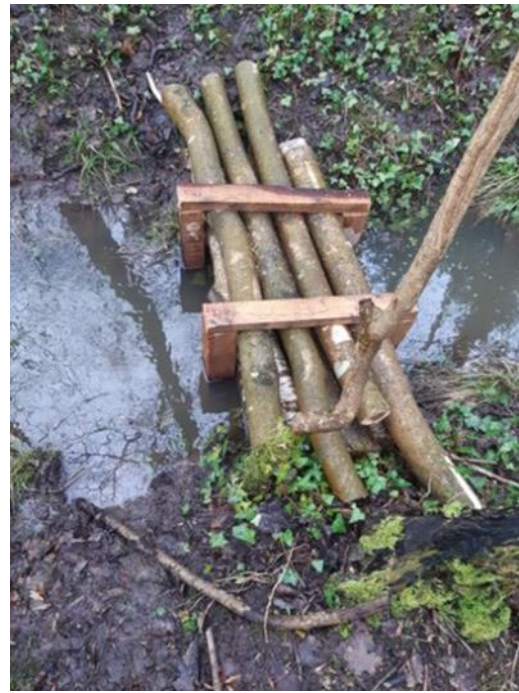
Timber logs from the estate have been utilised to create a secure leaky dam structure in channel to intercept nutrients and sediments. These installations also slow the flow backing up water increasing the potential for natural processes.
