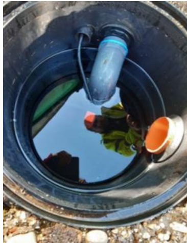
Left photo: downpipes make the most of the roof space. Pipes carry roof water to newly installed drain leading to new underground collection pit (right photo) and harvesting tank (below photo), which is connected to the irrigation system.
