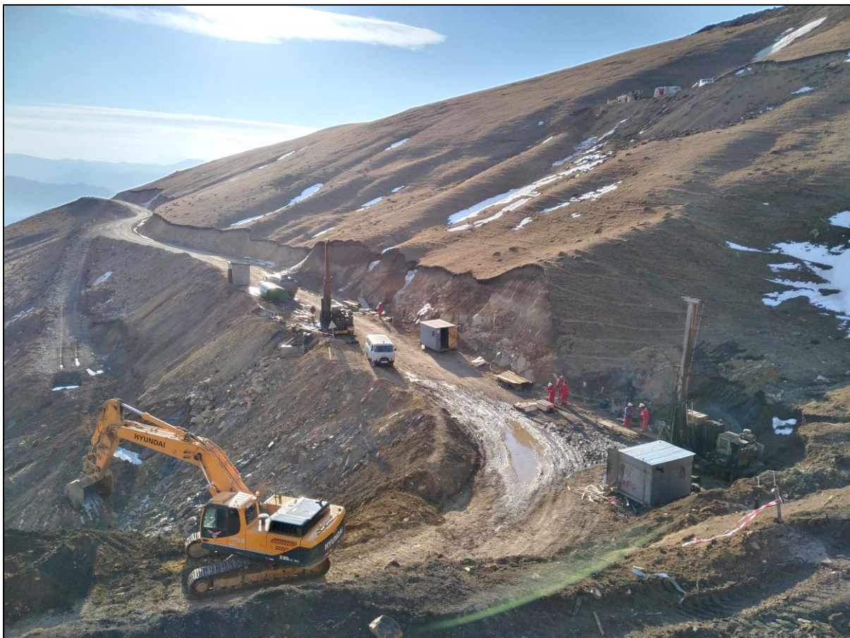
Figure 17 - Photo of Zafar drilling area. Looking to SW
