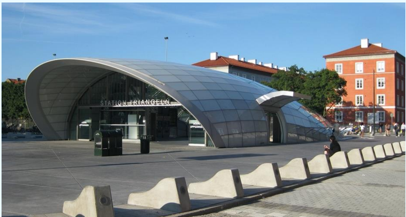
FIGURE 30 TRIANGELN STATION, MALMÖ SE - UNDERGROUND STATION (SOURCE: WIKIPEDIA)
