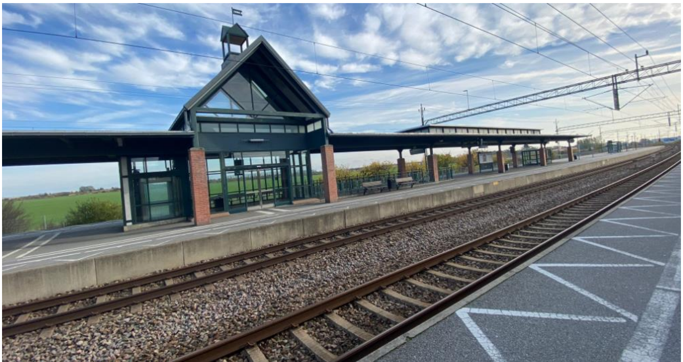
FIGURE 10 LANDSKRONA RAILWAY STATION, SWEDEN
