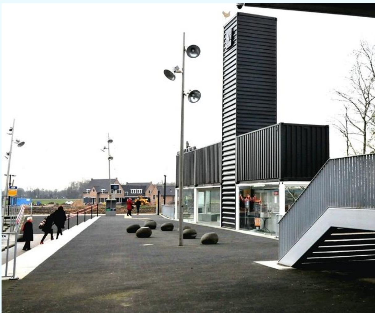
FIGURE 23 BARNEVELD NOORD STATION, NL – (SOURCE: WIKIPEDIA)
